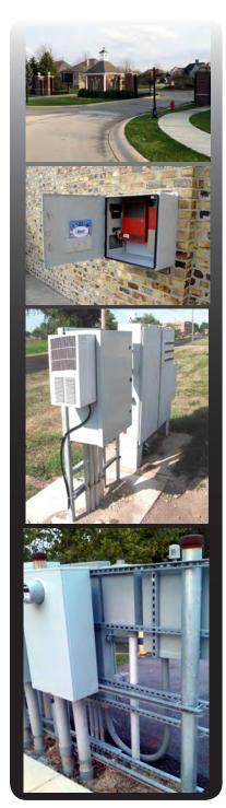
Along a gate using metal tubing to run wiring from one enclosure to another
